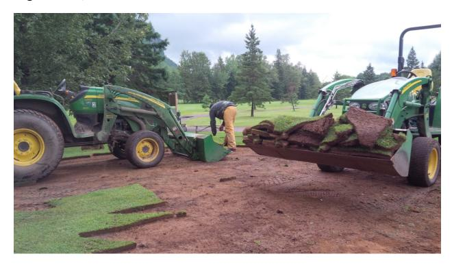
Existing sod stripped from deck. Two gator loads of sand and one load of soil incorporated into rootzone. Level area and sod with 750 ft2 of nursery tee sod. Topdress several times before September 8<sup>th</sup> opening.
