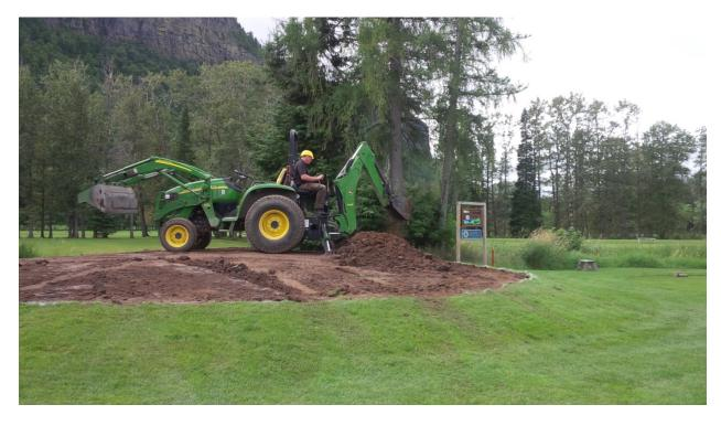
Material from trenching #12 fairway was placed at the backside of #8 black tee to lengthen the 188 yd hole to almost 200 yds. We shaved a foot off the top and pushed it to the back.
